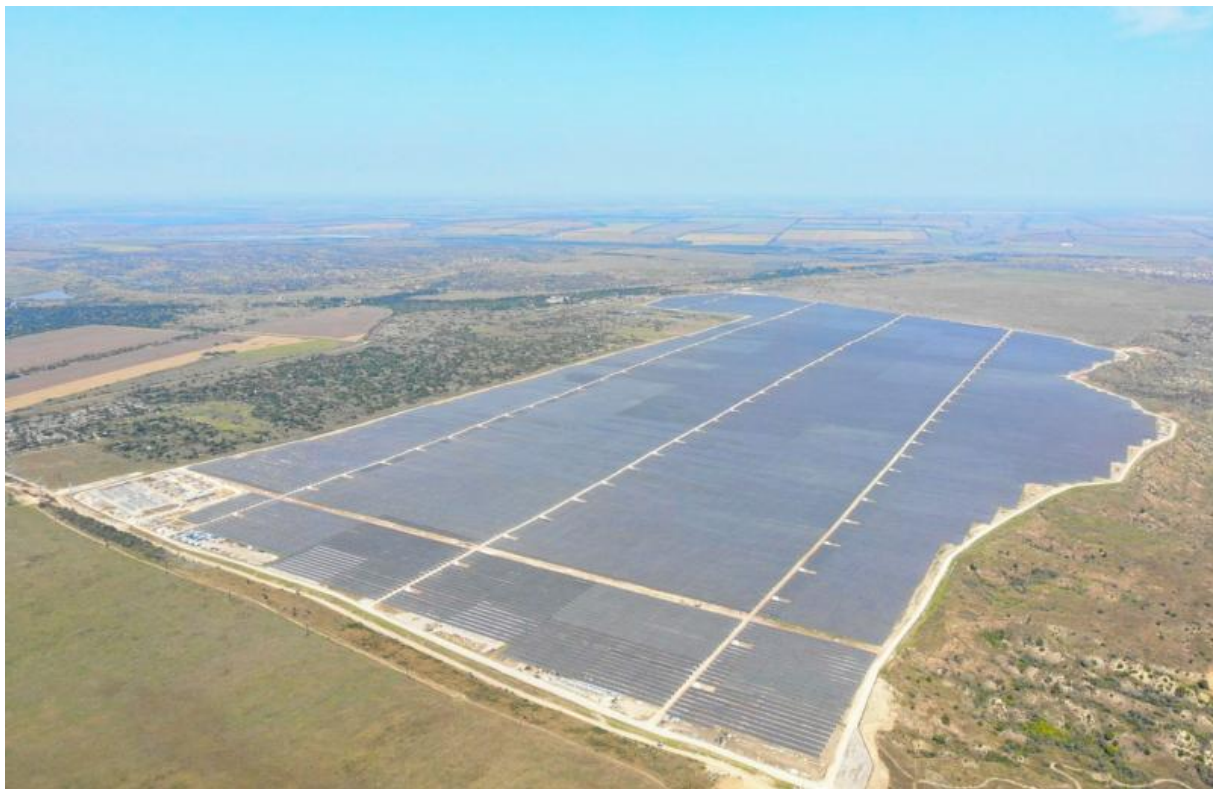
Figure 73. 240 MW solar power plant (source: DTEK)
