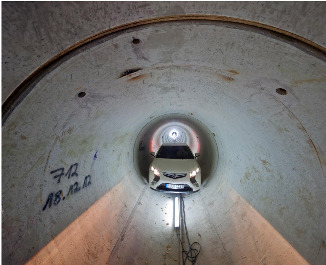
Figure 28. Car in new Emscher Sewage Canal (Source: Klaus Baumers / EGLV)
