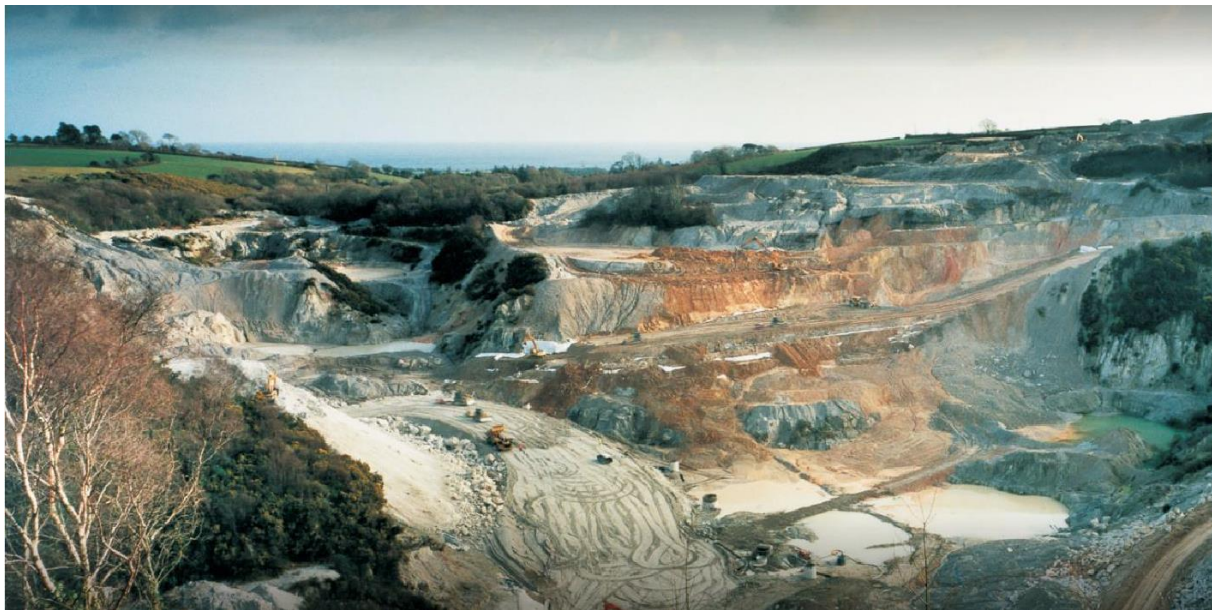
Figure 66. Bodelva pit right before Eden Project construction start
